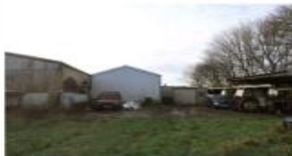
Figure 6: Rear view of farm buildings with western boundary.
